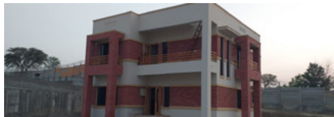
Constructed OrphanKind House
